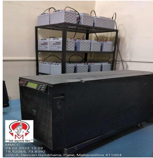
UPS with battery backup (20KV)
