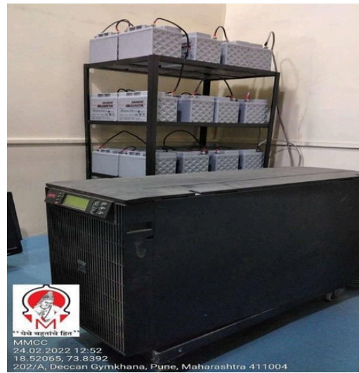
UPS with battery backup (20KV)
