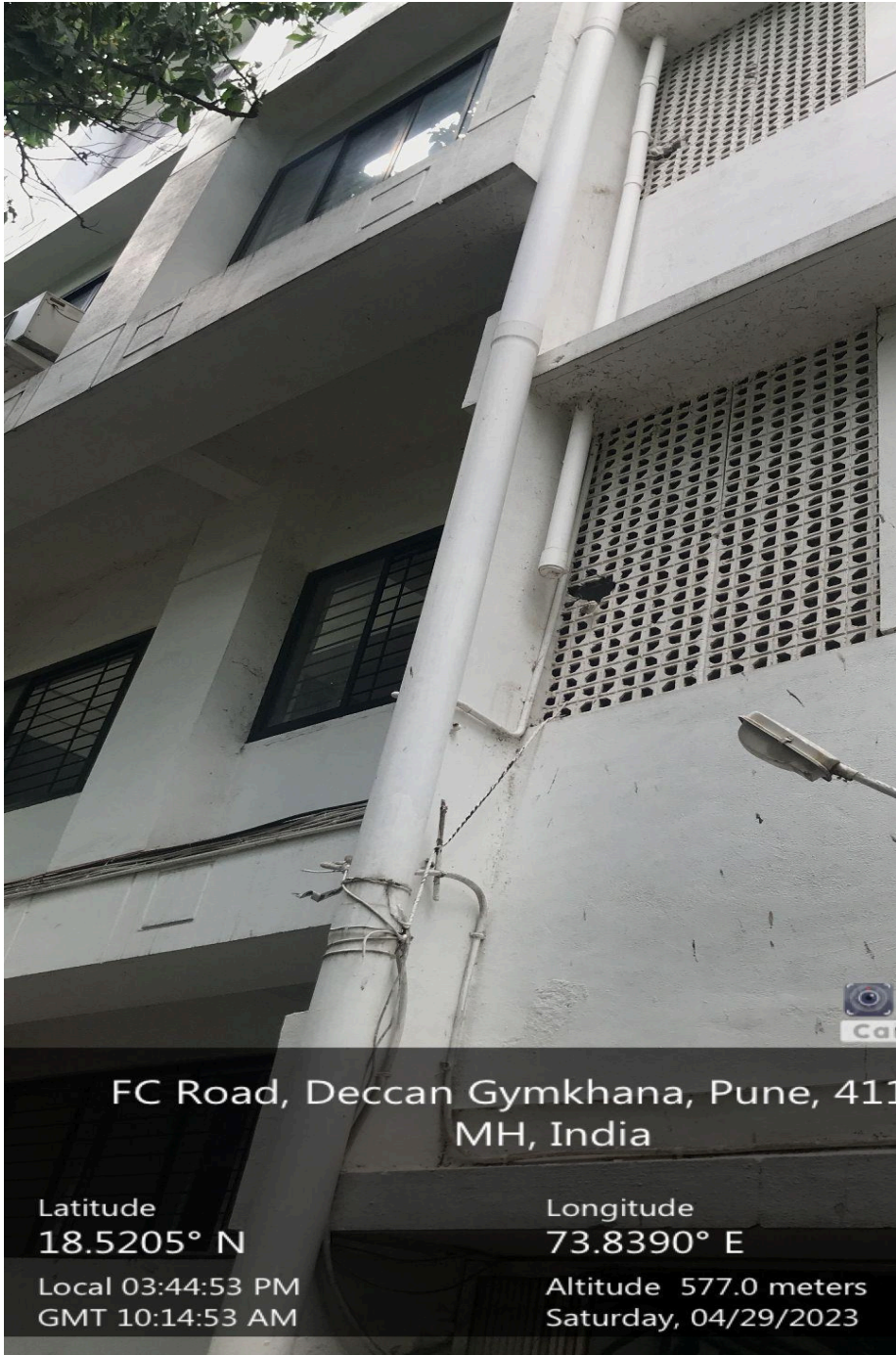
Rain Water Harvesting Channel-2
